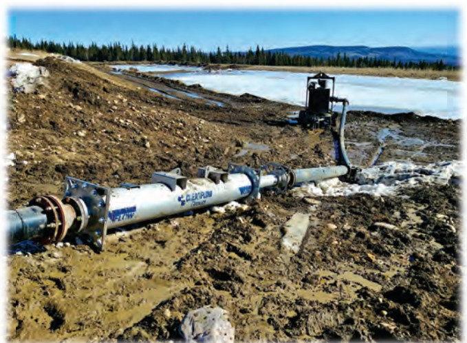
Pipe Reactor installation at Westmoreland Mountain mine location
